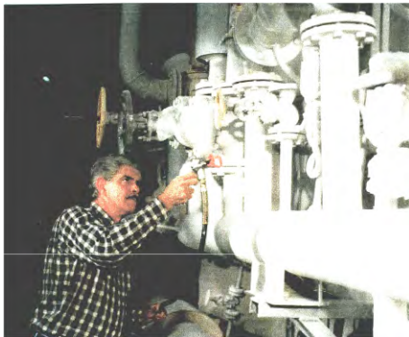
Piping easily coated with airless spray
