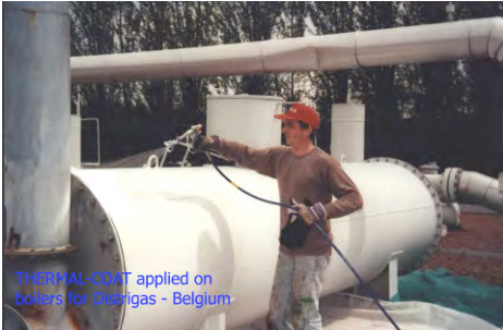
Coating Distrigas Boilers
